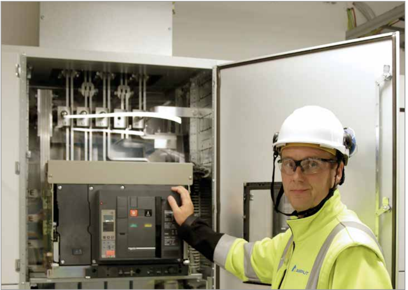
The new children's hospital - The busbars for the Children's Hospital were designed and manufactured by Lapp Connecto, and installed in July-August 2017. The hospital environment poses special demands for magnetic fields around busbars.
